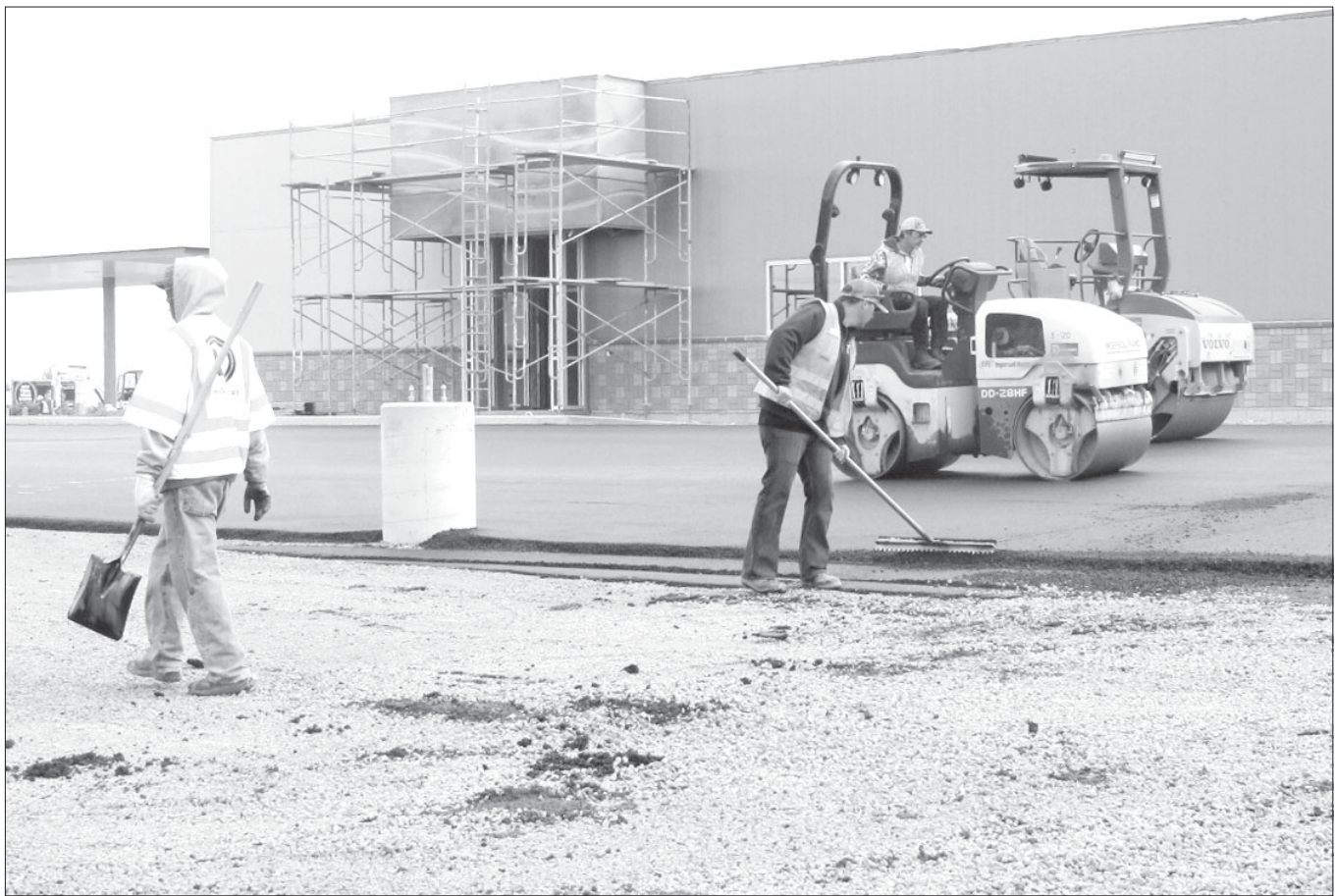
The construction crew puts down the asphalt paving at the Plateau Travel Plaza.
