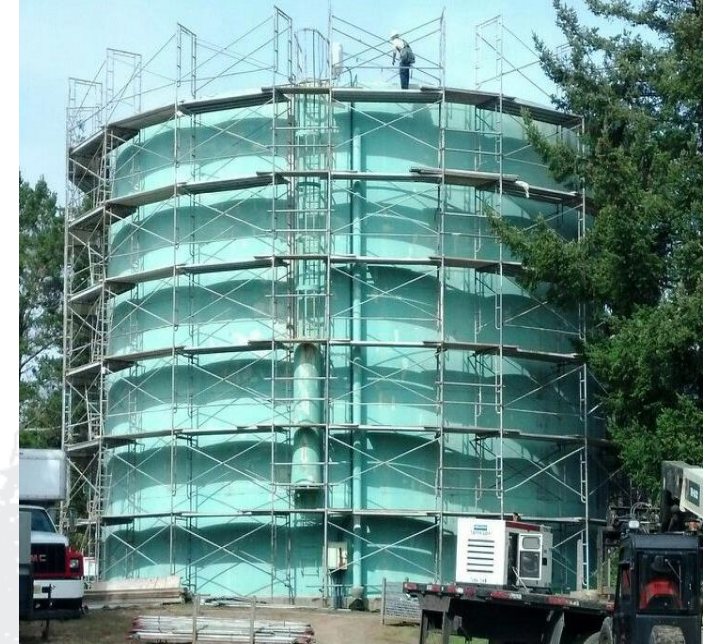
Reservoir Tank Recoating
